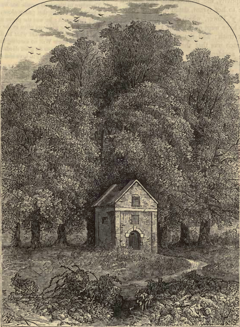
OLD CONDUIT, GREENWICH PARK, IN 1835.
