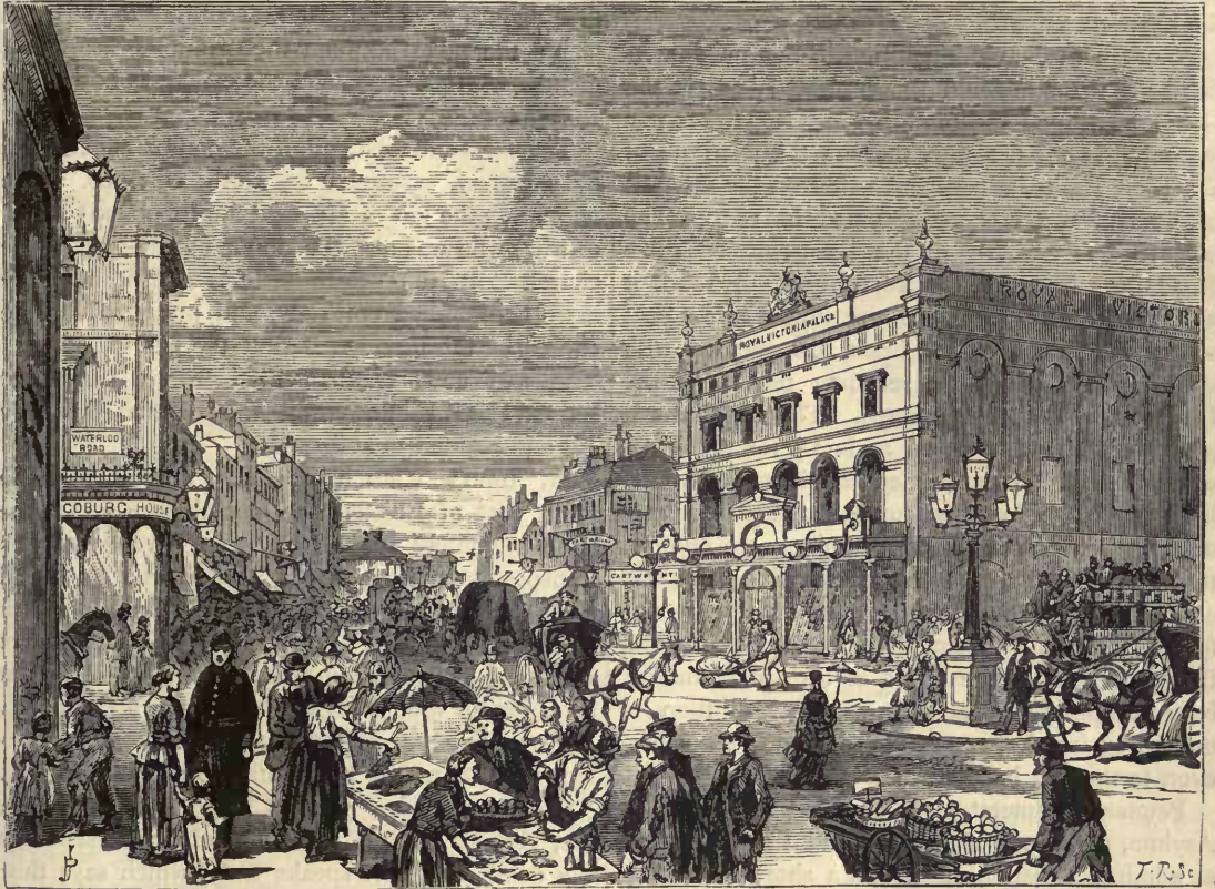
VIEW IN THE NEW CUT.
