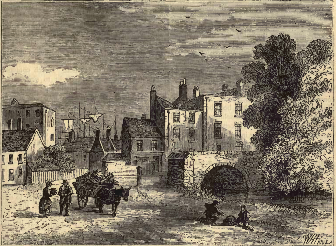
MILL POND BRIDGE, IN 1826.
